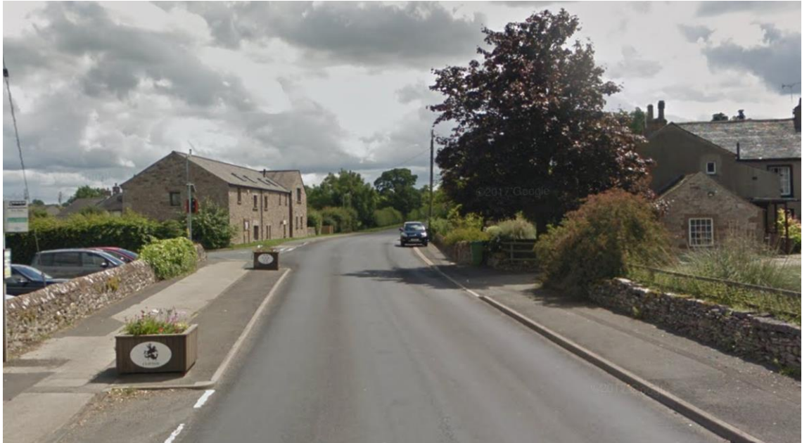
Figure 14: Carriageway narrowing and no centre-line on A6 at Clifton in Cumbria
