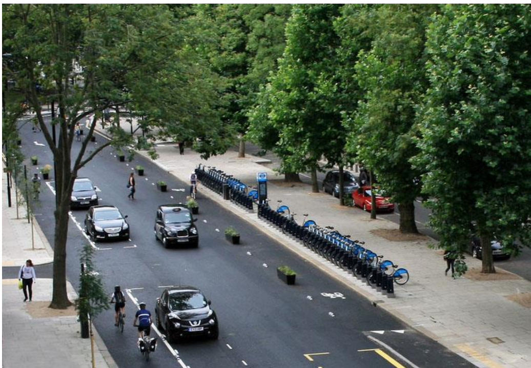
Figure 11: “Floating parking bays” and reduced road width create cycle lane and reduce speed
