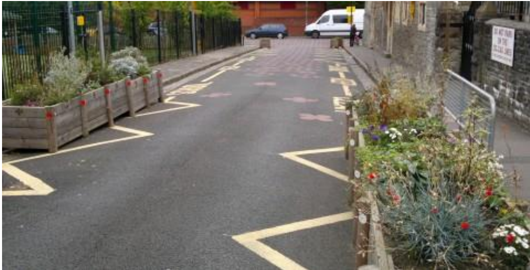
Figure 10: Planters placed in carriageway to discourage stopping outside school and reduce speed
